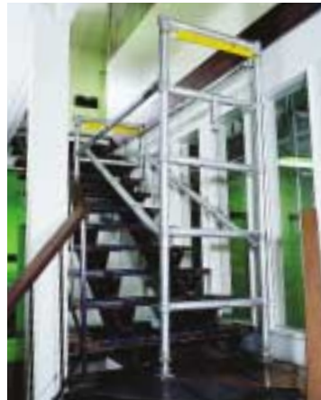
Set up base section on stairway.
