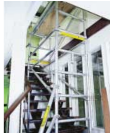
Add aluminum extensions, platforms, guardrails and toeboards plus outriggers, if required.
